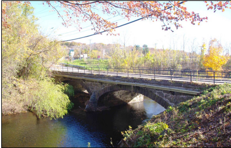
Figure 3.10.3 Glover Avenue Bridge (Bridge No. 4135), looking southeast.
