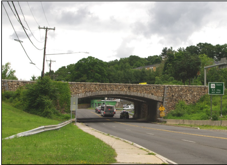
Figure 3.10.4 Main Avenue Bridge (Bridge Nos. 560A and 560B), looking north.
